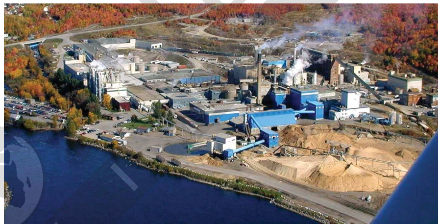
Tembec produces food-grade ethanol at its Tamiscaming, Quebec, Canada site using specialty pulp from the facility as a feedstock. Photo courtesy of Tembec.
